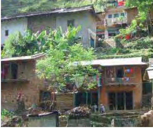
Mijhing Runiban ( Ch. 0+000)Starting point
