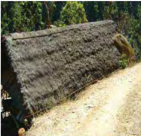
Affected House at Ch. 2+020 (Badachaur VDC)
