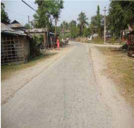
Existing blacktopped road at Ch 4+ 100
