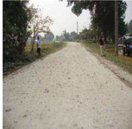
Existing road at Ch 4+200, road width is 6m
