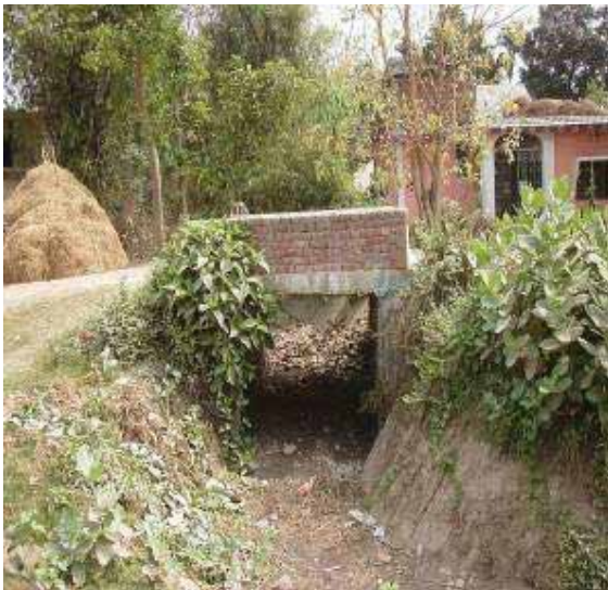
Irrigation crossing at Ch. 5+744
