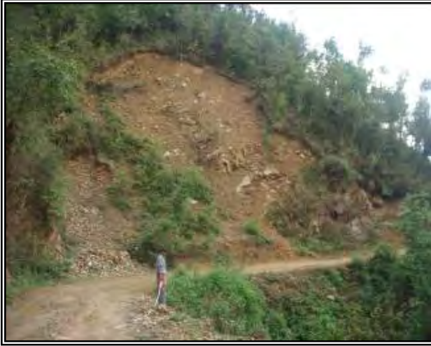
Road alignment along landslide area.
