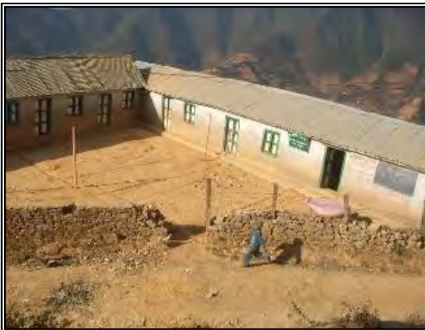
Photograph showing project affected public structure
