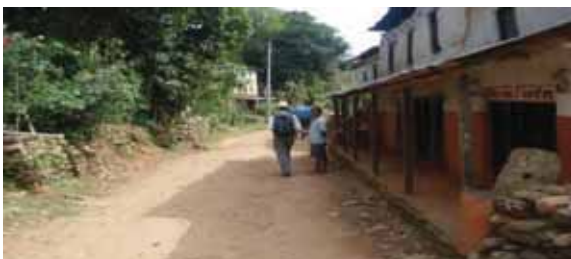
need resettlement work at chainage 13+200
