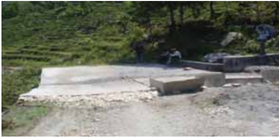
Existing PCC causeway at chainage 1+760
