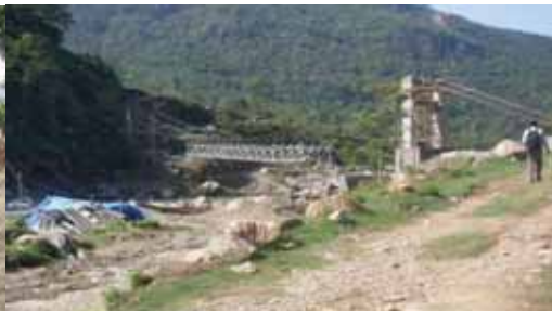
Moterable Suspension Bridge on the road alignment at chainage 0+860
