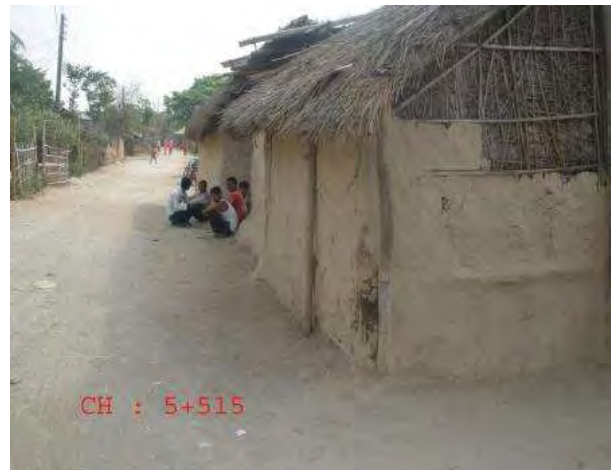
Affected Small hut at Ch. 5+515
