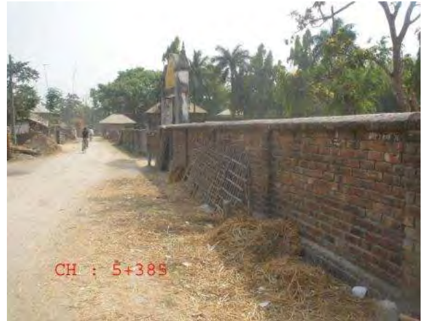
Affected Boundary wall and gate of school at Ch 5+385
