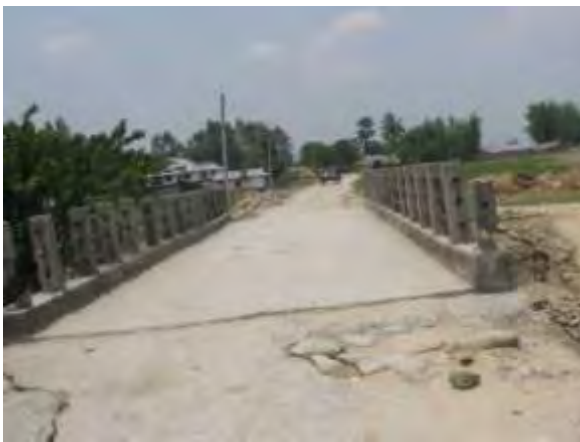
Dhadhara Khola Bridge (Ch 8+855)
