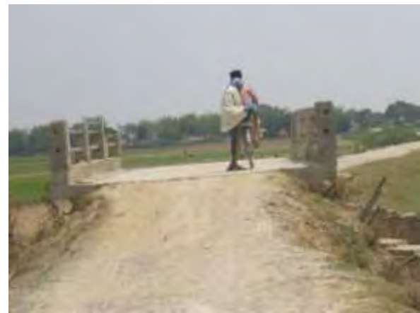
Pahara Khola Bridge (Ch 3+264)
