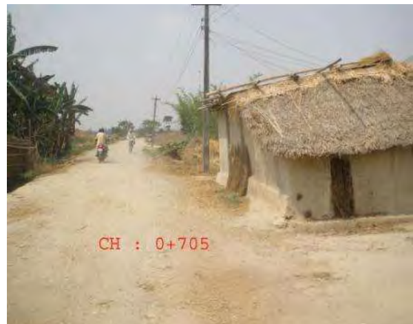
Affected house at Ch 0+705
