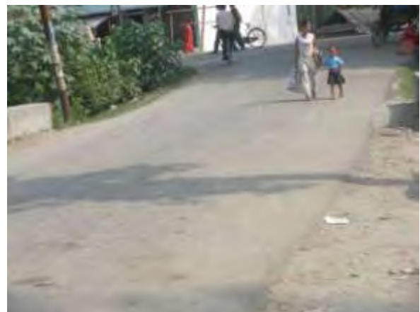
End of Road (Pathari VDC Ch: 30+900)
