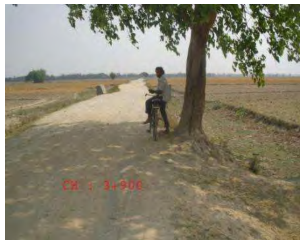
Affected Peepal tree at Ch 3+900
