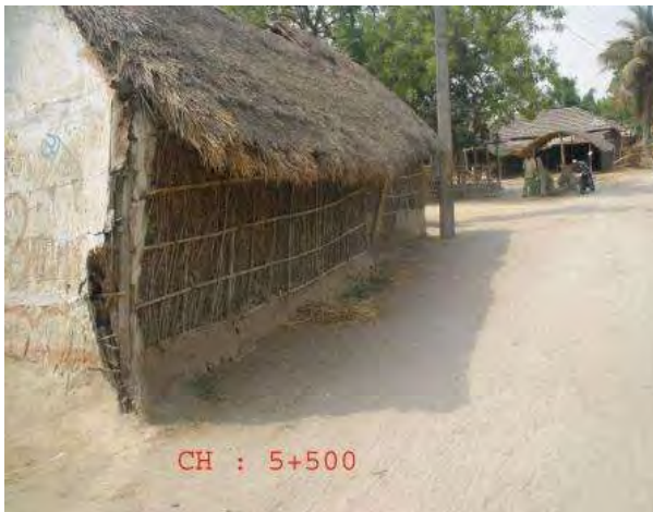
Affected Small hut at Ch. 5+500
