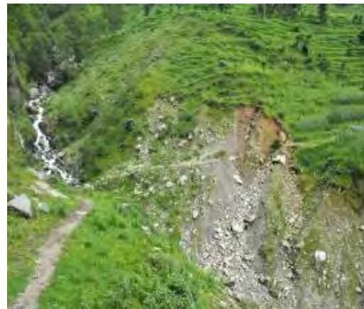
Jethal Khola (Ch 4+750) : Minor slide area along the alignment
