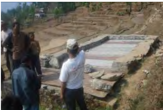
Water Tank at Ch 11+985
