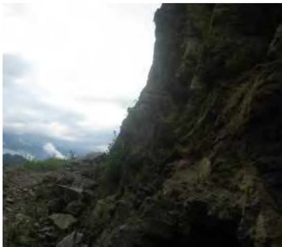
Exposed rock along the alignment at Ch 4+980
