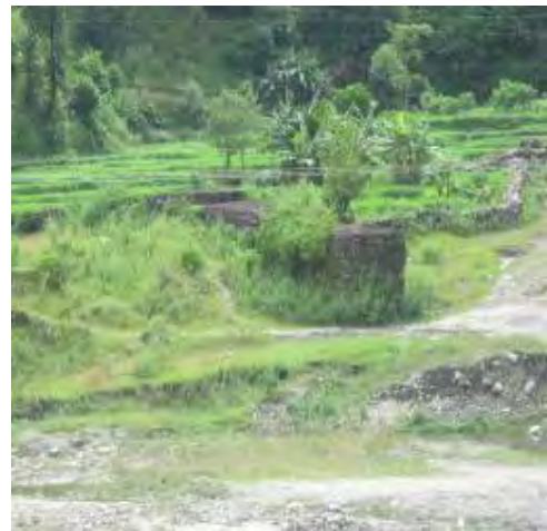
End point of the alignment at Damsite, Balka (Ch 22+921).
