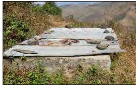
Common Property: Reservoir Tank (Ch 1+720)
