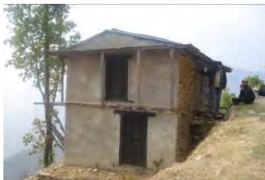
House at Ch 14+540
