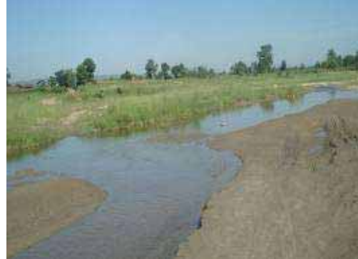
Parayu Khola crossing the road at (Ch17+990) which requires protection work.
