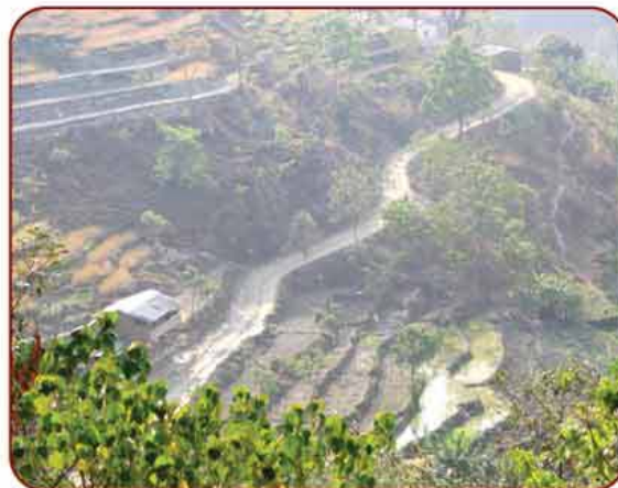
Baglung-Burtibang Rural Road at Khahare Baglung
