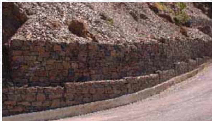
Hill side protection work and side drain: Shenal to Saunel Road, Length: 4.28 Km., Cost- 125 Lakhs, District Shimla, Himachal Pradesh.
