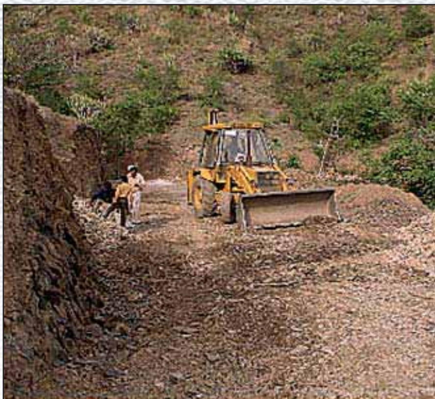
Hill side cutting for construction of formation of the road, Danughat to Kolka Road, Length:2.5 Km., Cost-62.83 Lakhs. District Solan, Himachal Pradesh.
