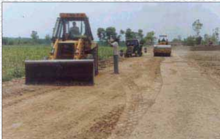
Compaction of the sub-grade soil of the road, Rampur Fakhruwal to Rampur Road, Length 2.47 Km., Cost Rs 40.55 Lakhs, Year 2001-02, District Jalandhar, Punjab.
